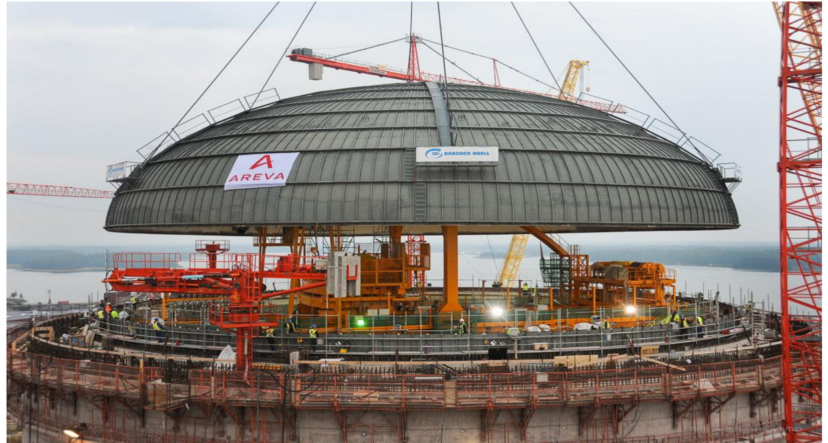
Fabrication and supply of steel containment liner OL3 Project – new EPR unit in Nuclear Power Plant in Olkiluoto.
